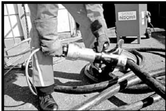
Cutting of cable.
