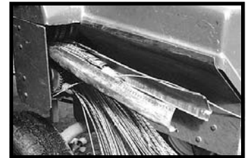
Easy stripping of lead covered telephone cable.
